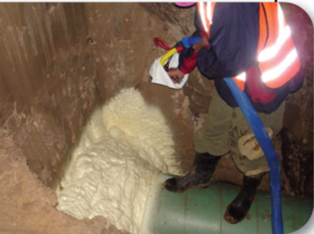
^ TerraThane can be installed quickly without scorching or foam splitting.
