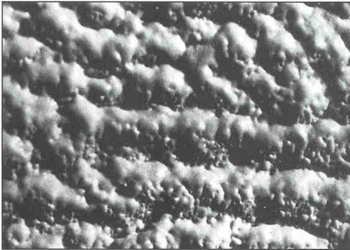
Photo 4 Polyurethane Foam Texture Rippling – Verge of Popcorn
